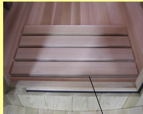
Duckboard Floor Section
